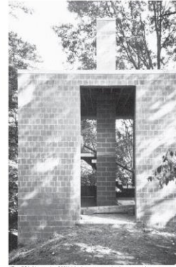
(Fig. 11) Above, the CMU blocks are turned sideways to show variation in the course pattern.
