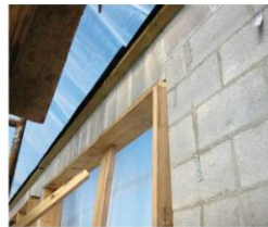
(Fig. 10) Reinforced literals are used to span window and door openings in walls. Above, the CMU blocks are turned vertically so rebar can be set horizontally through the cavities.
